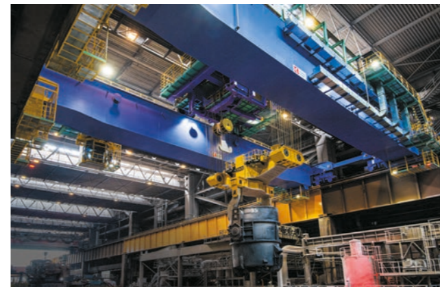
Pfannentransportkran 390/60t x 40m ©Foto: thyssenkrupp Steel Europe AG
